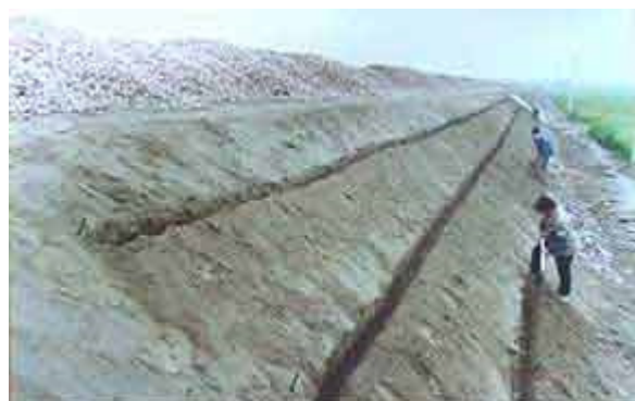
Preparing small planting trenches along embankment. .... Newly planted vetiver
