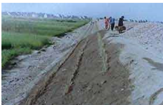
Preparing small planting trenches along embankment. .... Newly planted vetiver
