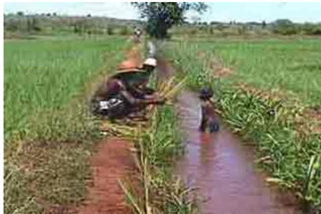
Member of water user association planting vetiver grass along canal bank
