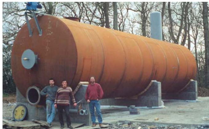
Figure 3 The first digester under construction.
