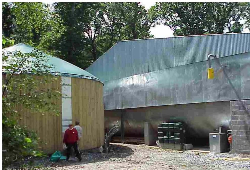
Figure 7 The plug-flow digester (right of picture) and the continuously stirred digester with biogas storage (left of picture).
